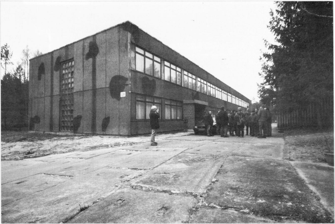
The main peacetime entrance to the 3 level bunker is from the adjacent HQ building
